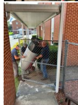
New water heater going downstairs
